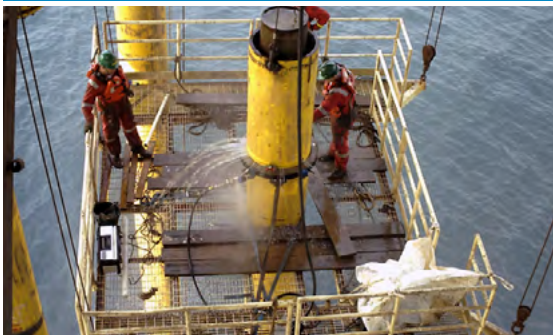
TT762 Cutting and beveling machine with pneumatic drive
